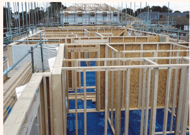
Image of off-site manufacture, courtesy of Willmott Dixon: www.willmottdixon.co.uk
