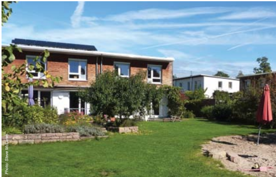
Passivhaus 'Building Group' at the Smiley Barracks Project in North Karlsruhe, Germany - The city council set up an arms-length development management company to assist 10 'building groups' realise this 195 home scheme, for a range of income groups and special needs; all to high environmental standards.
